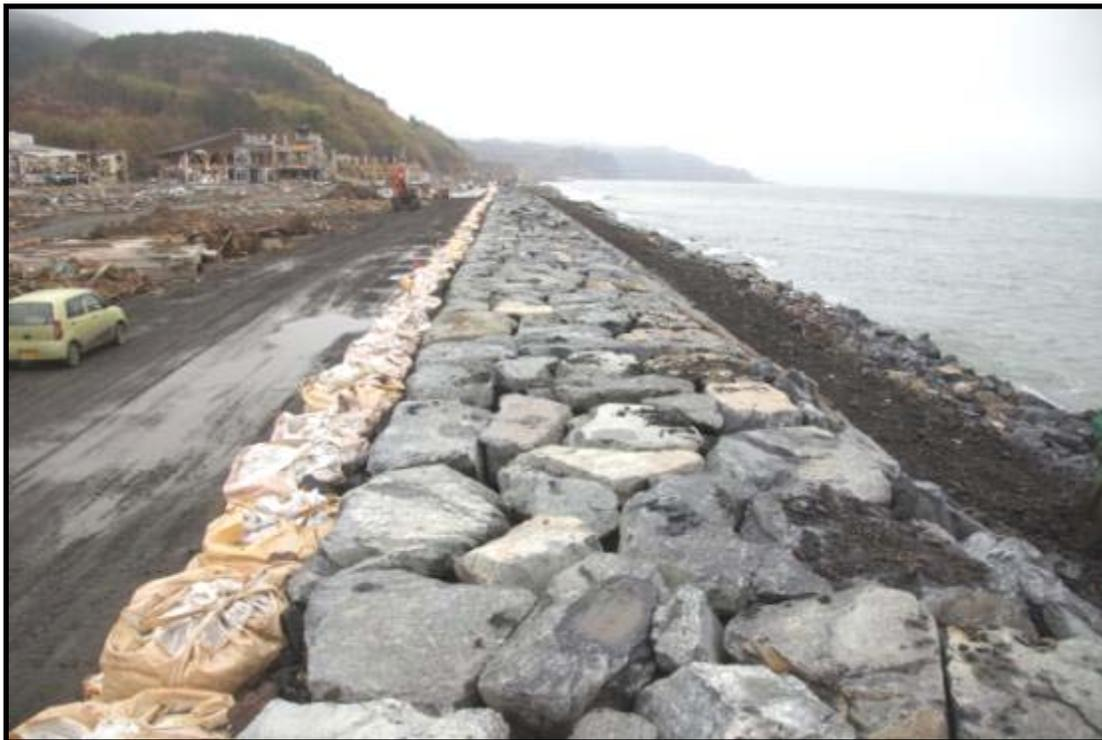
Figure 25: Photographs of Construction Equipment Being Used to Provide Interim Flood/Tsunami Protection Along Left Kitakami River near River Kilometer 0.5 (N38.5739, E141.4498, April 22, 2011)
