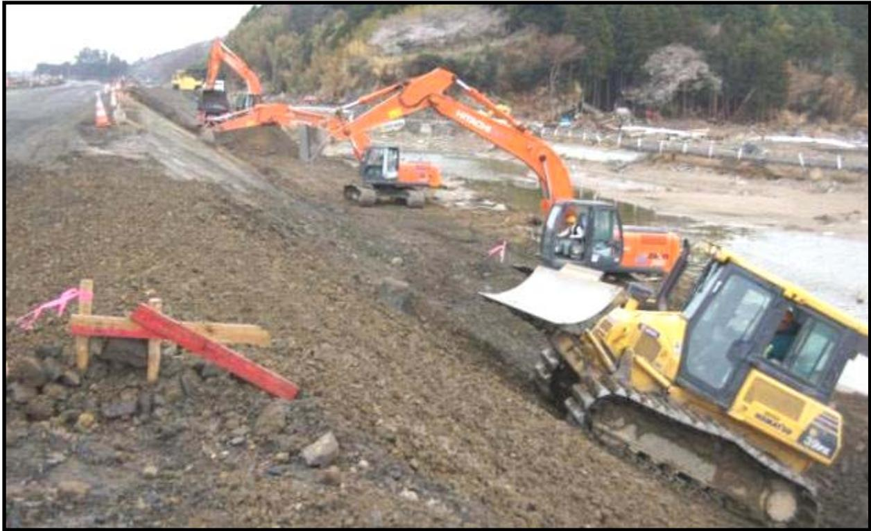
Figure 24: Photograph of Construction Equipment Being Used to Rebuild Landside Levee Section Eroded Along Left Kitakami River Levee by Tsunami Waves near River Kilometer 1.5 (N38.5703, E141.4384, April 22, 2011)
