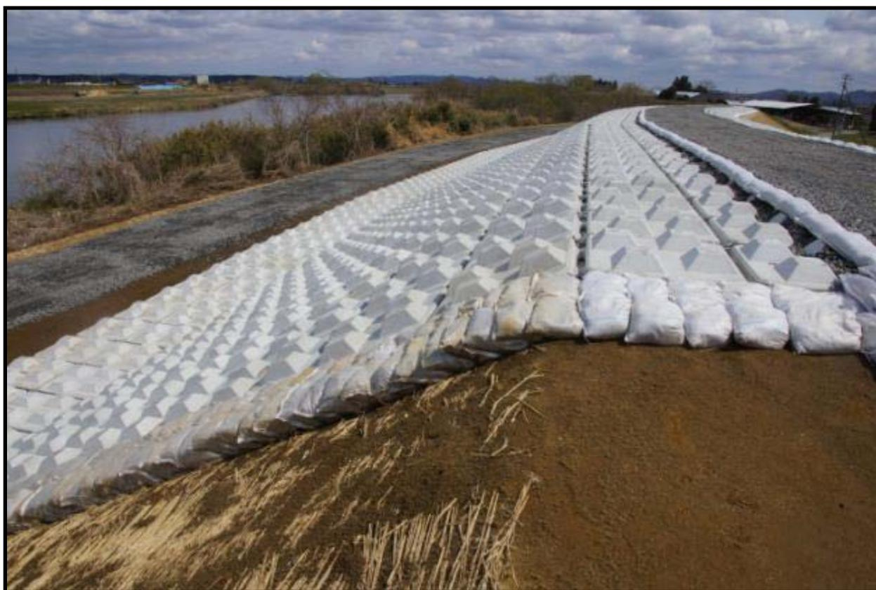
Figure 12: Completed Interim Repair of Liquefaction-related Damage to Naruse River Left Levee at River Kilometer 11.3 (N38.4538, E141.1087, April 21, 2011)
