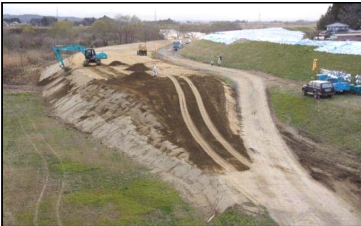
Figure 9: Photograph of Construction of Large Waterside Berm as Part of an Interim Repair of the Naruse River Left Levee at River Kilometer 30.1 (N38.5333, E 141.0050, April 20, 2011)
